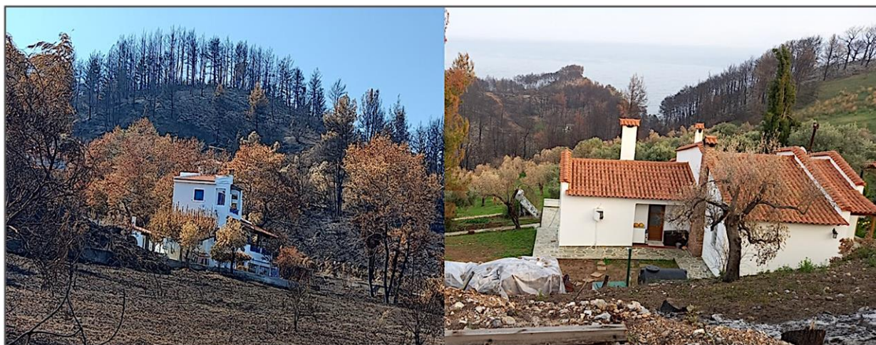
Figure 1. Houses with minor damages due to the construction material and existence of defensible space
