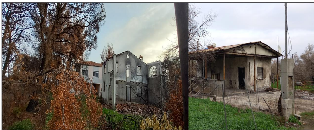
Figure 2. Houses with significant damage due to pure or aged construction materials
