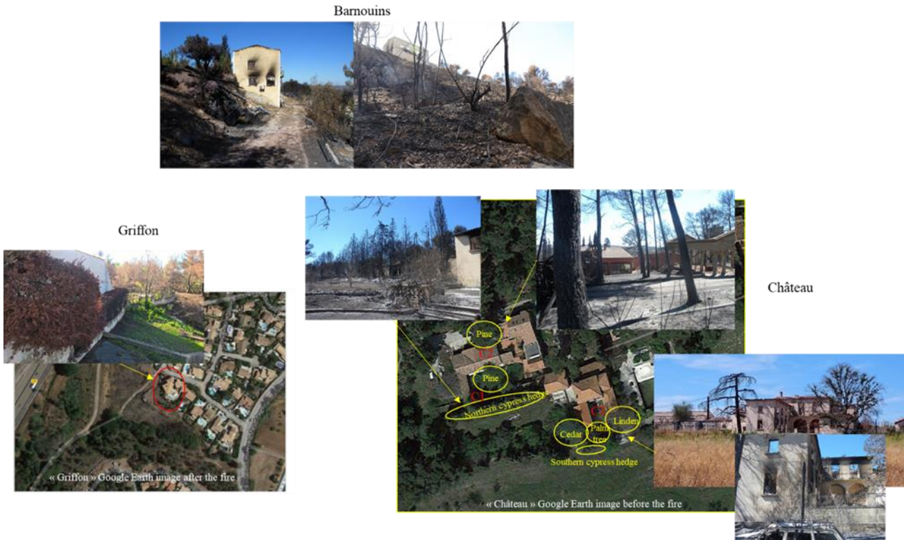
Figure 3 – Pictures of the post-fire damage recorded in the three study cases.
