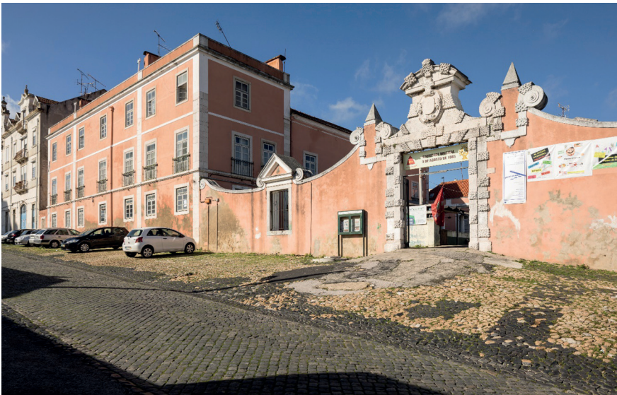
Figure 4: Marquês de Abrantes Palace in Marvila street, Lisbon. Source: Ateliernob / Francisco Nogueira, 2017.
