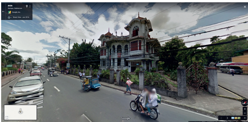
Figure 2: Street view showing the Natalio Enriquez mansion and its enclosing fence and gates made of wrought iron, brick and concrete (Google, 2016).
