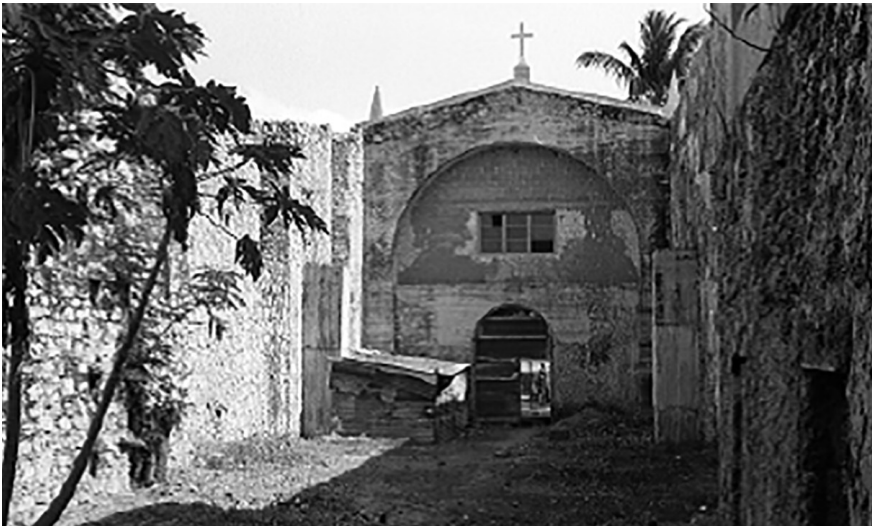
Figure 11: Interior of S. Domingo's Church under reconstruction, 1983.[Services].
